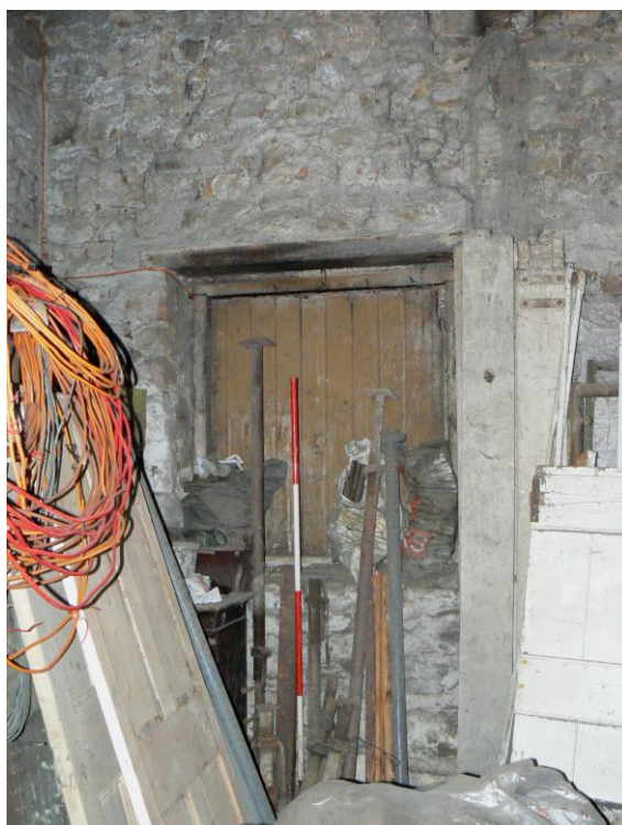
Plate 10: Hatch (13) in the west wall of the barn
