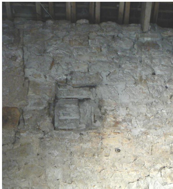
Plate 12: Blocked opening (7) in the south wall
