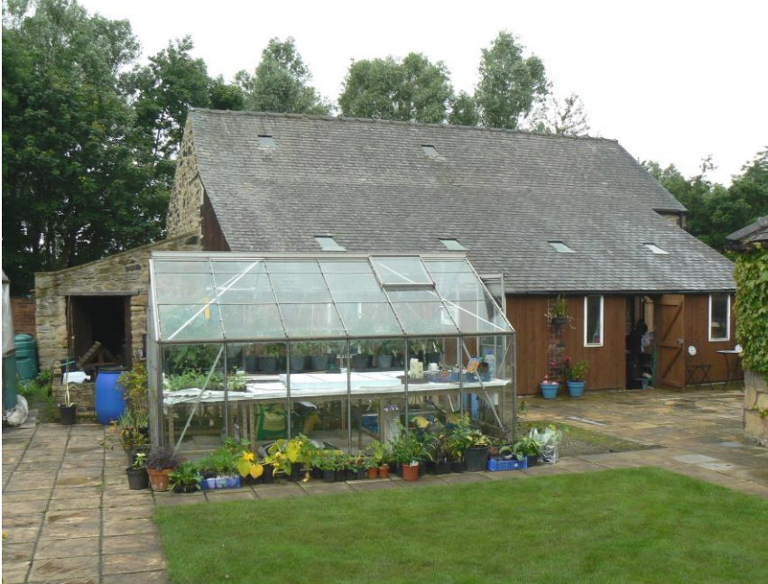
Plate 4: Greenhouse and timber addition to south wall of barn
