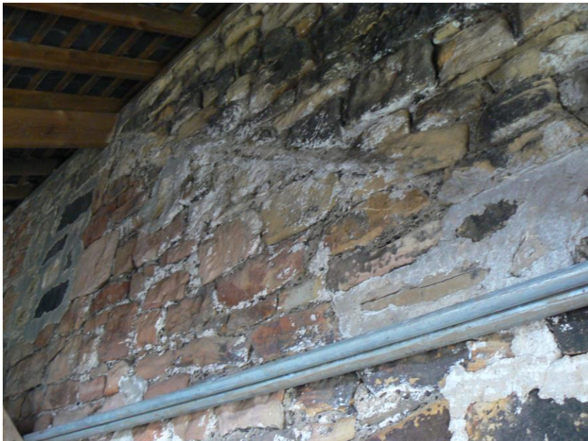
Plate 6: Scar of gin gang gable on external face of south wall of barn. Note the reddened burnt stone within the scar
