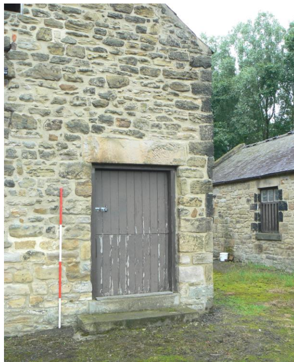
Plate 8: Door in the east wall (14)
