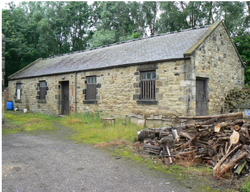
Plate 14: Stable block (B) to the north of the barn. Looking from the south-east
