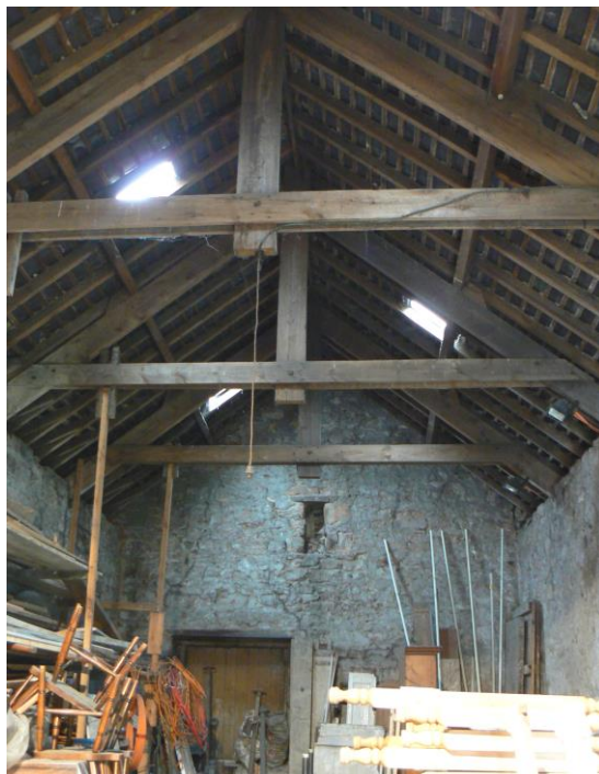
Plate 9: The roof structure of the barn
