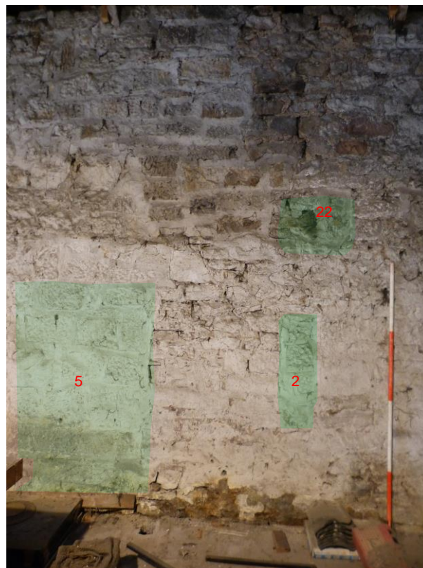
Plate 2: Inner face of south wall of barn. Blocked entrance [5] towards centre. Features toned in green and numbered as per catalogue
