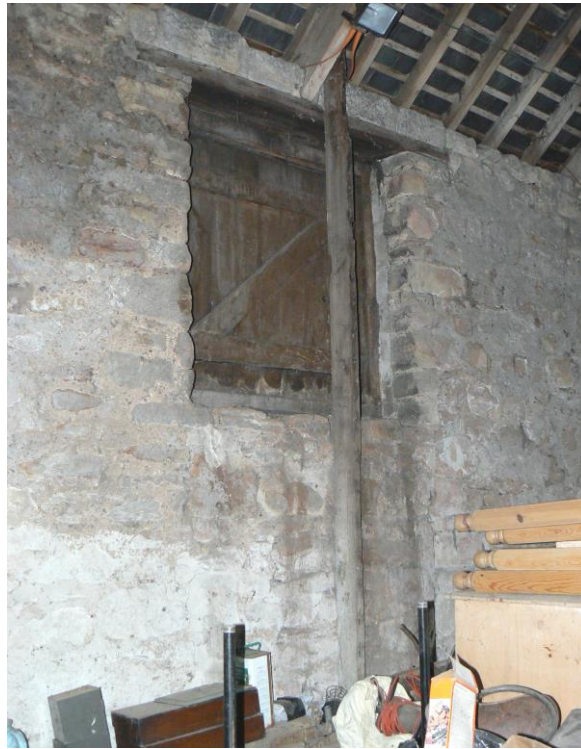
Plate 11: First floor pitching door (11) in the north wall
