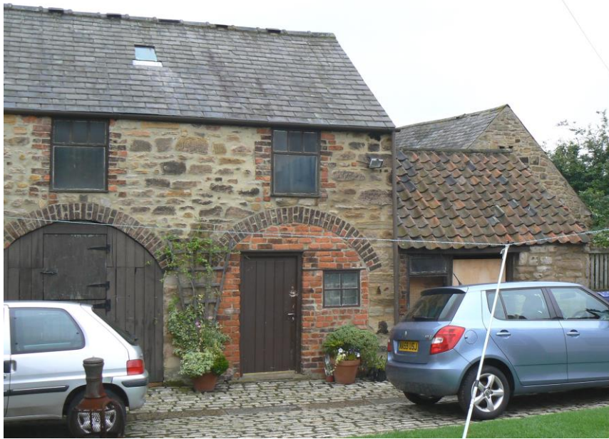
Plate 15: The southern part of Cart shed (C) from the west
